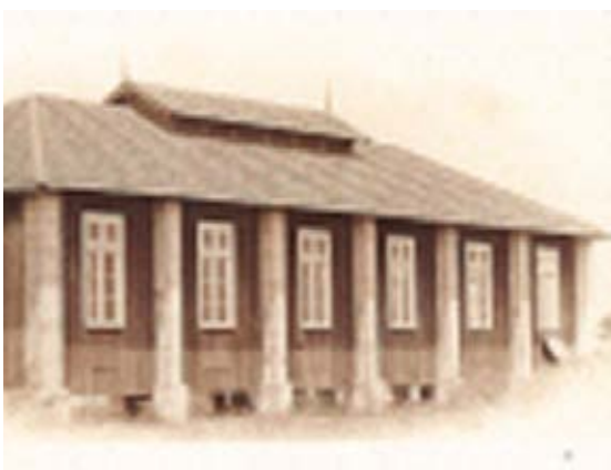
Figura 5: Hospital Goelas de Pau
